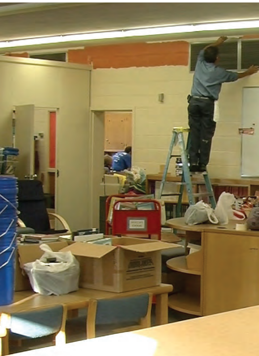
WFMY Team renovates Media Center at Sedgfield Elementary
