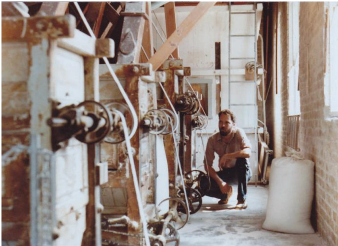
North State Milling Company Building interior, c. 1975.
