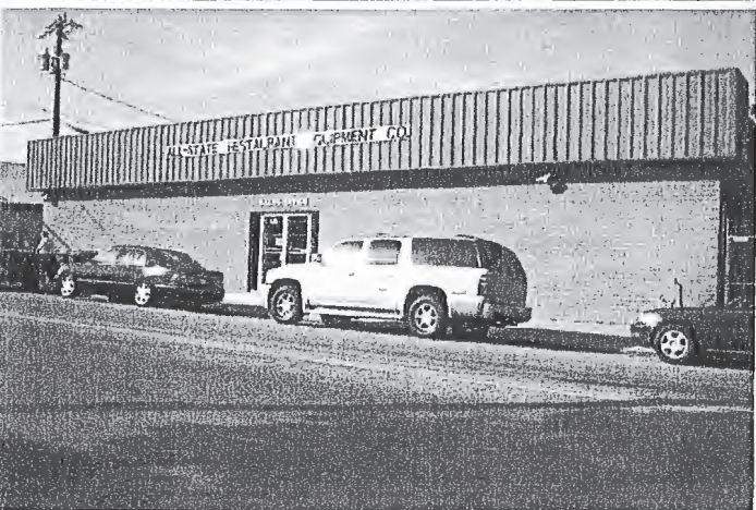
870 S. Elm St All-State Restaurant Equipment Co.
