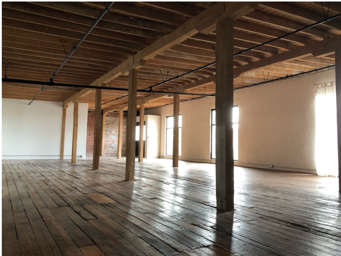
Interior of mill soon after adaptive reuse. Historic materials retained on floors, columns, walls, ceilings, and beams.
