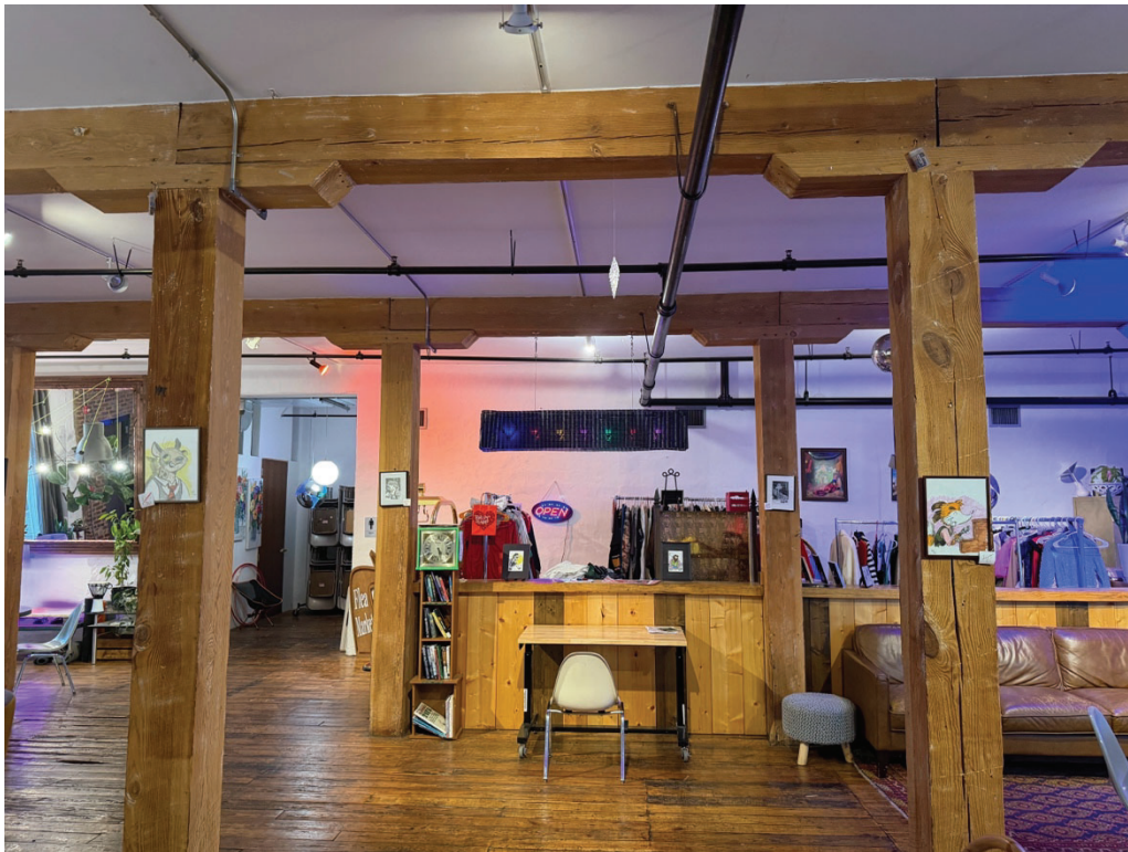
Photo 6: 1965 addition, facing west. Wood support beams, columns, floors are retained.
