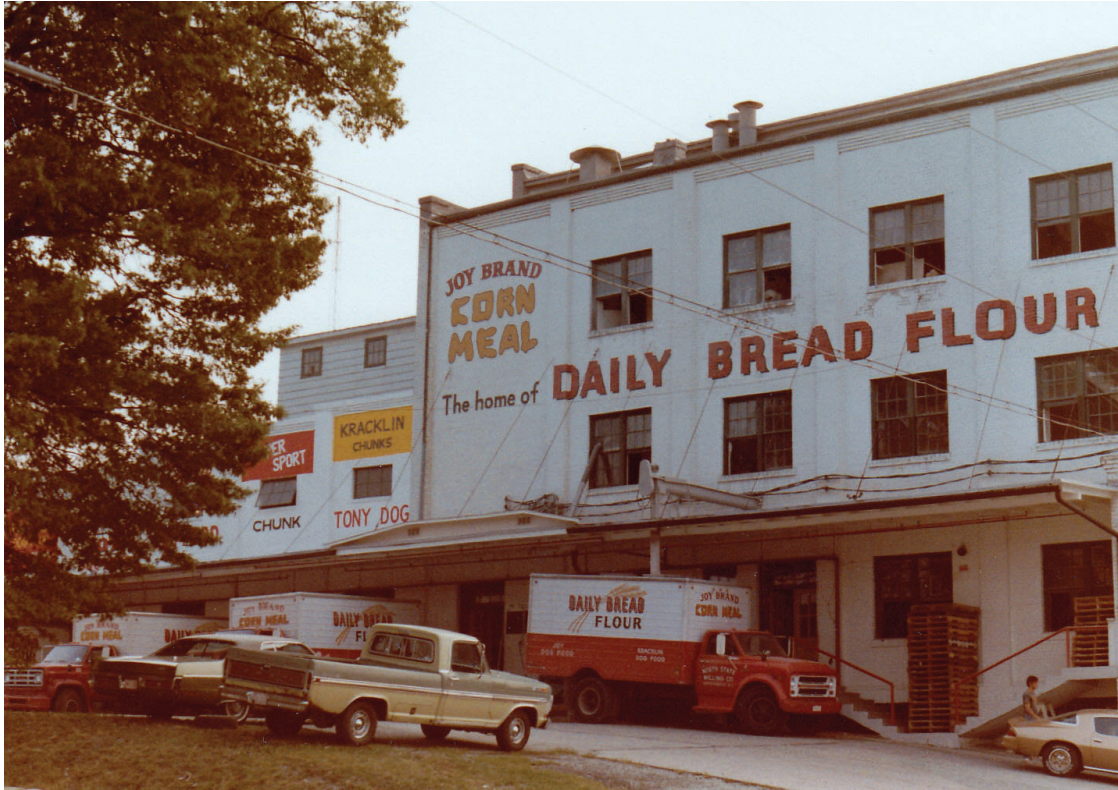
North State Milling Company Building east elevation, c. 1975.
