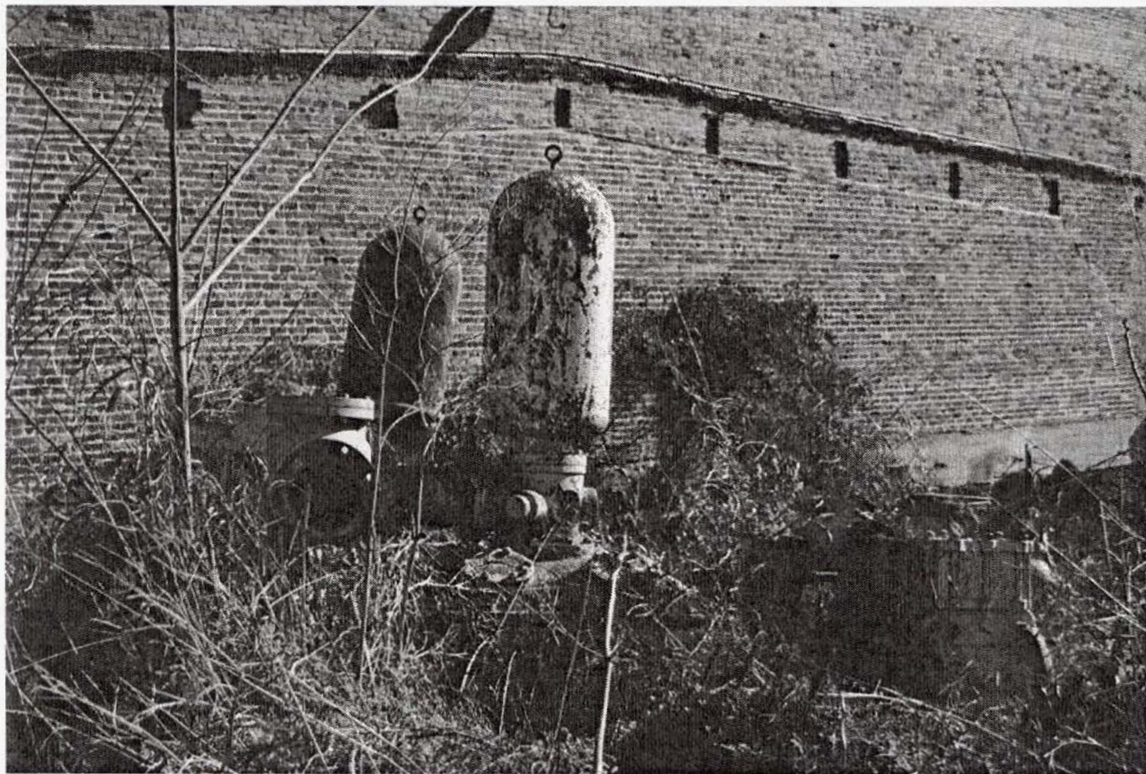
p.138 - Building I, west facade, former intermediate firewall, between bays.
