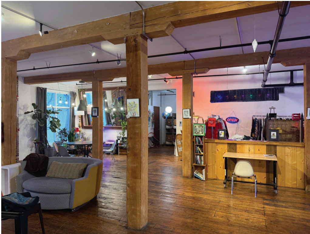
Photo 6: 1965 addition, facing west. Wood support beams, columns, floors are retained.
