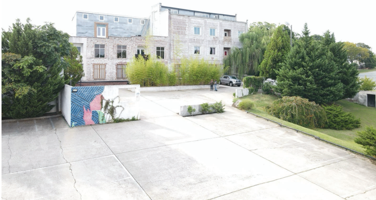
North State Milling Company Building, east elevation, c. 2014.
