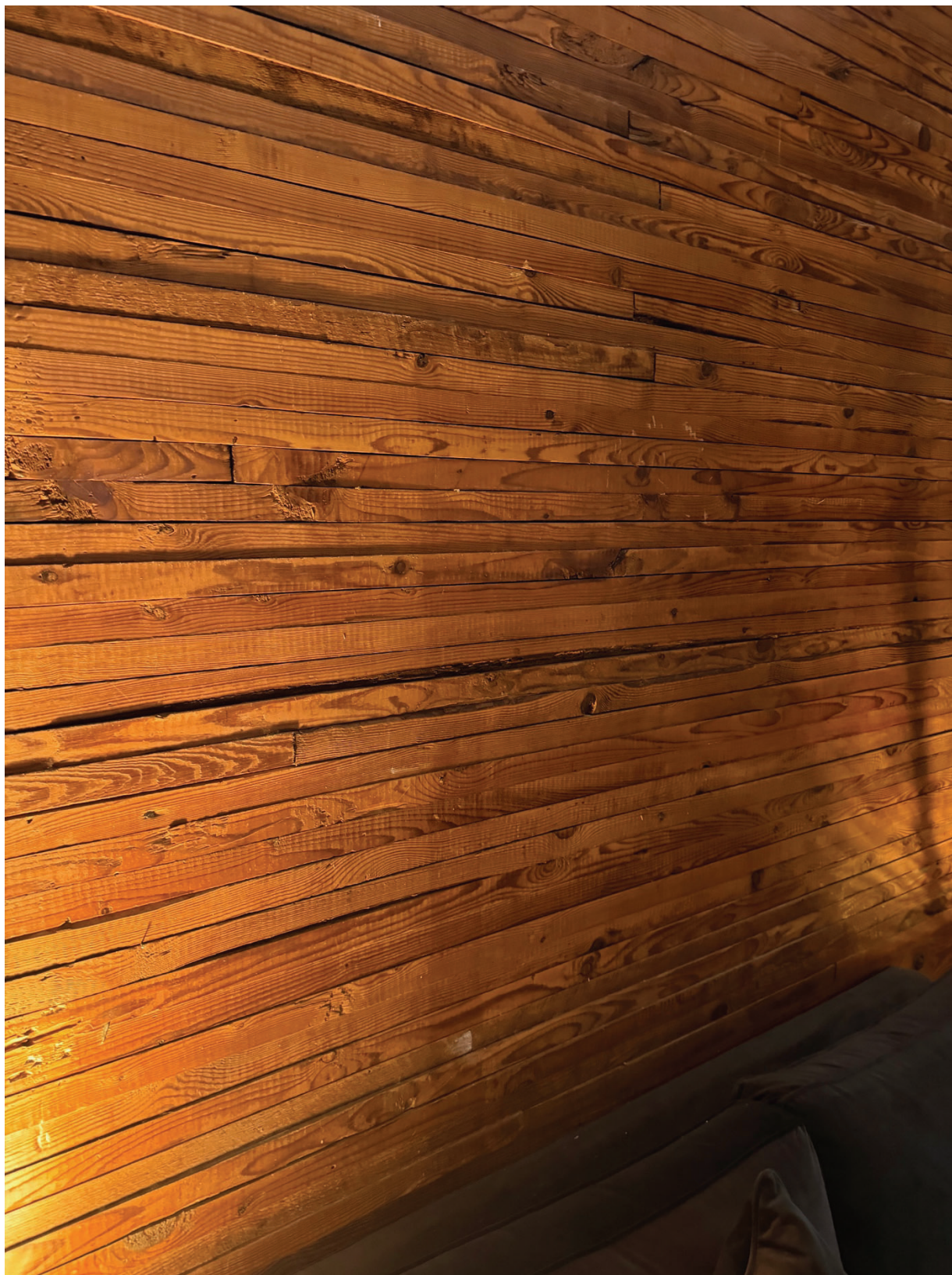
Photo 6: Interior silos retained.
