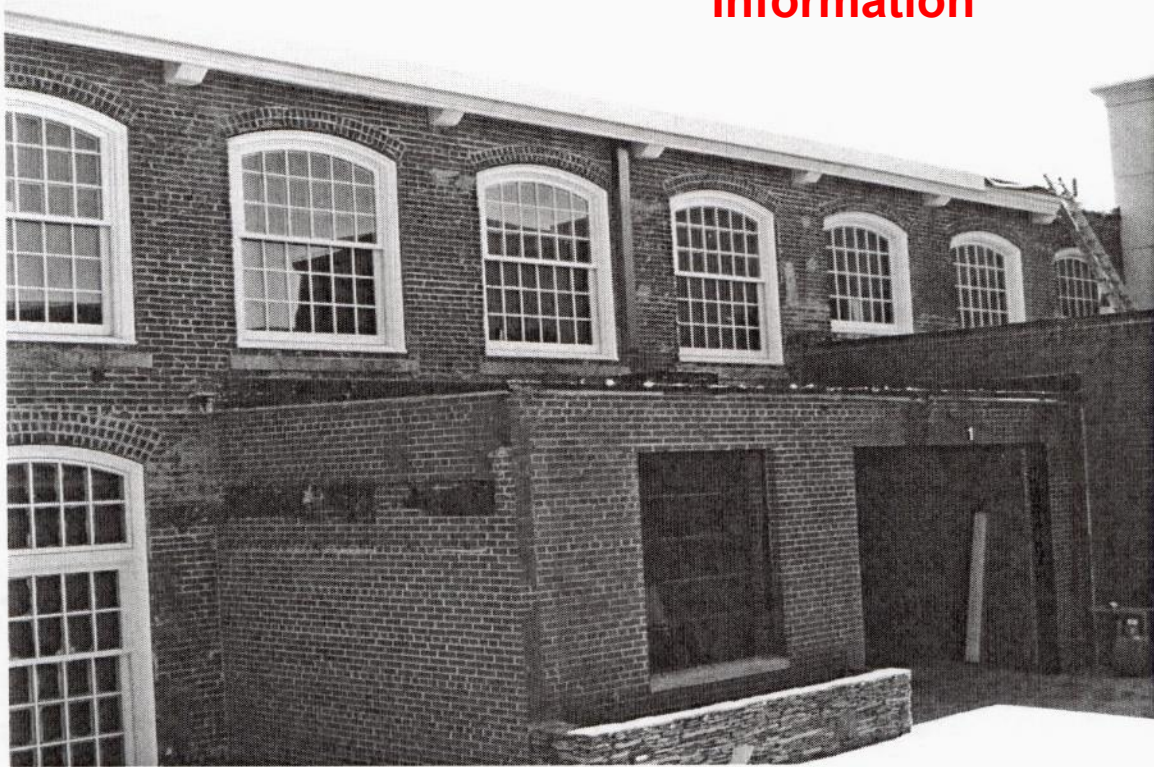
p.133 - View looking southwest. Building E, north appendage addition.
