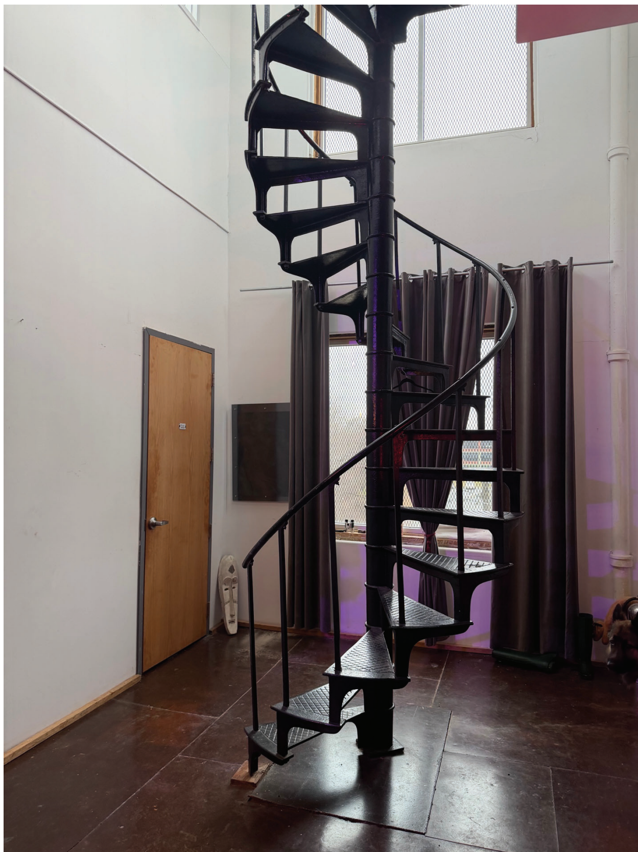
Photo 6: Metal stair installed at the north end of the 1912 main block.
