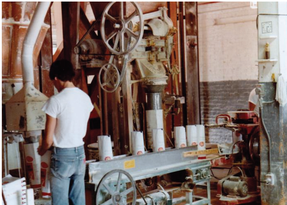
North State Milling Company Building interior, c. 1975.
