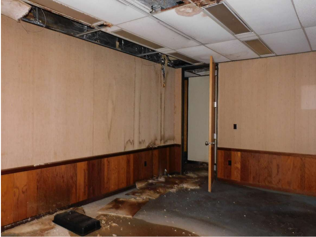
Figure 12: Detail of the wall finishes and deteriorated conditions on the 8th floor.
