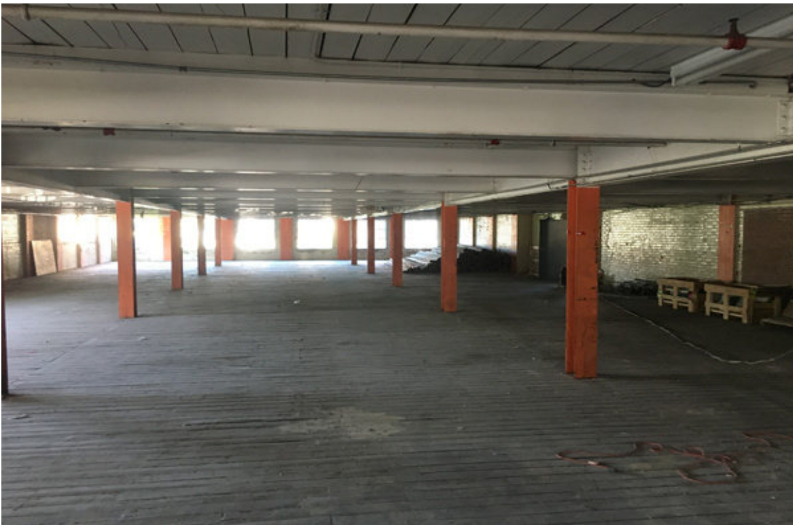
p.18 - 1st floor building interior of the 1930 warehouse addition Looking South showing steel structure & wood floor decking between the first and second floor.
