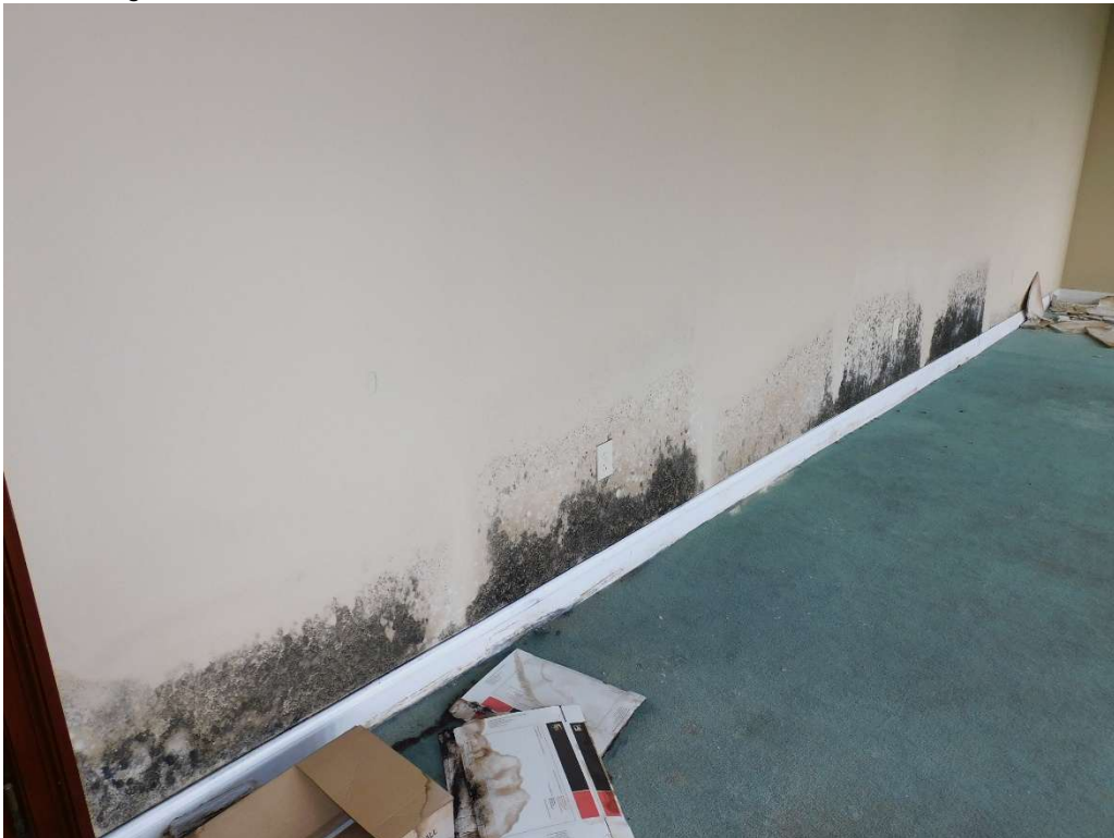
Figure 13: Detail of mold growth on walls of 8th floor.
