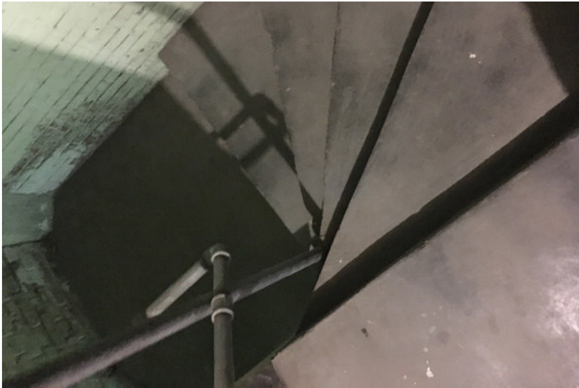
p 19 - East stair tower between first floor and mezzanine level showing the winder treads to be modified.
