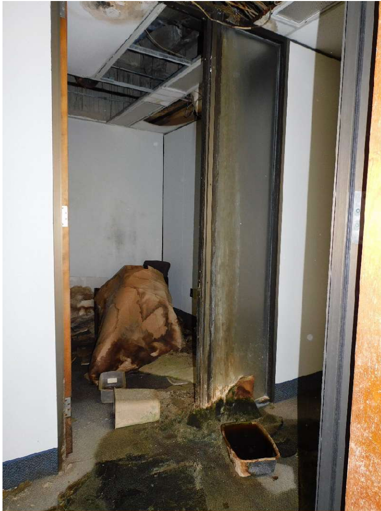
Figure 10: Image showing typical wall and ceiling condition on the 8th floor.
