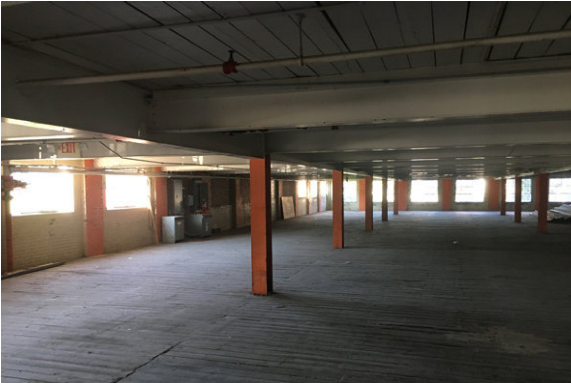
p.17 - 1st floor building interior of the 1930 warehouse addition Looking South West showing steel structure & wood floor decking between the first and second floor
