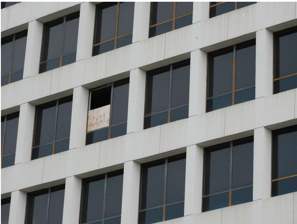
Figure 8: Detail showing example window boarded over.
