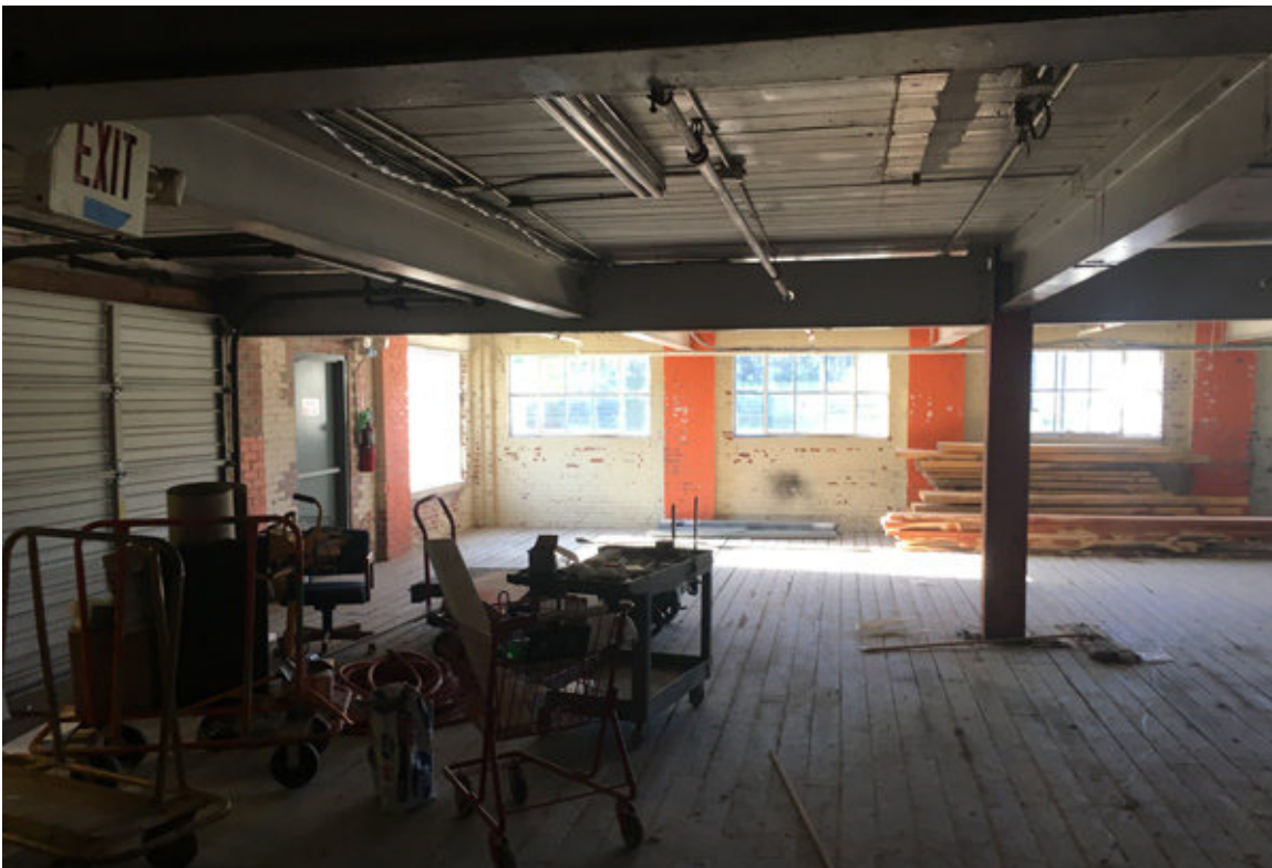
p.16 - 1st floor building interior of the 1930 warehouse addition Looking South East showing steel structure & wood floor decking between the first and second floor.
