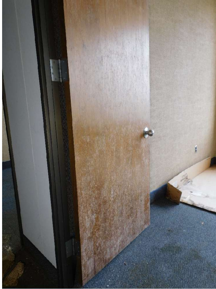
Figure 14: Door detail showing mold growth on 8th floor.
