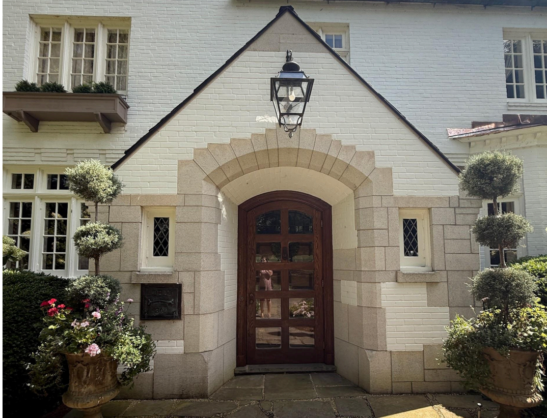
Image 20: Main entrance exterior
