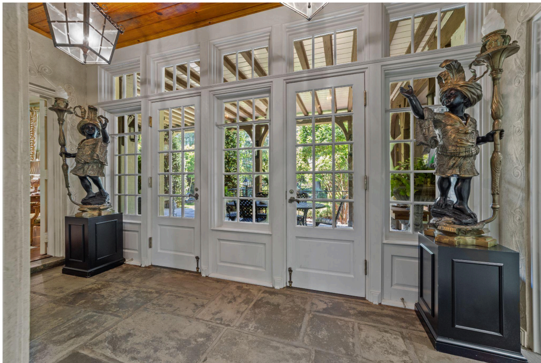
Image 37: Interior view of the original 3/4 lite french doors and transom windows.
