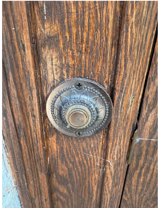
Image 22: Detailed view of the main doorbell.
