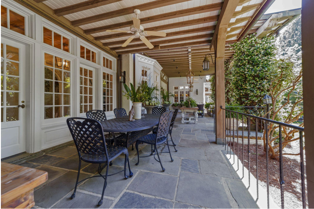
Image 38: Exterior view of the original ¾ lite french doors and transom windows.
