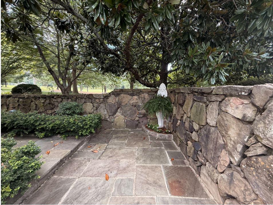
Image 28: Walkway to secondary entrance.
