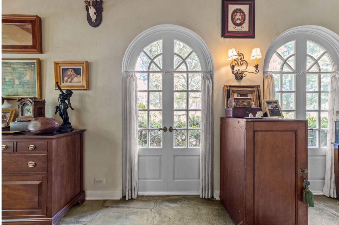
Image 40: Detailed view of the arched french door with a divided fan lite above.
