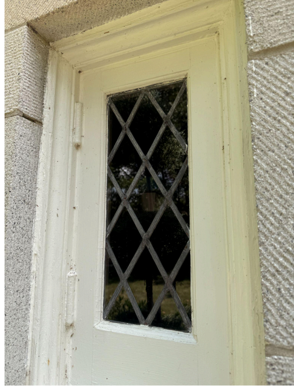
Image 24: Detailed view of sealed casement windows of the main entryway.
