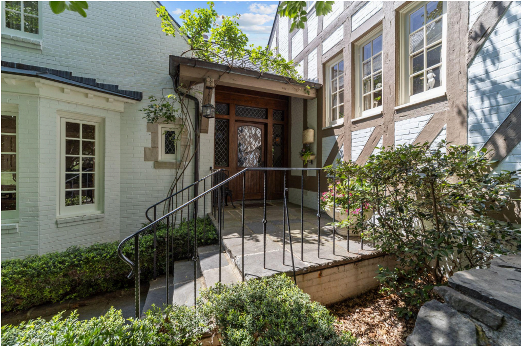
Image 30: Secondary entrance exterior
