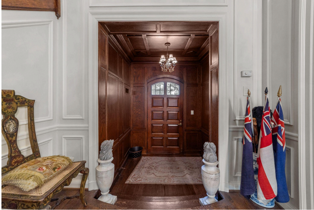
Image 26: Main entrance interior showing the interior side of the 8 paneled ¼ lite solid wood door.
