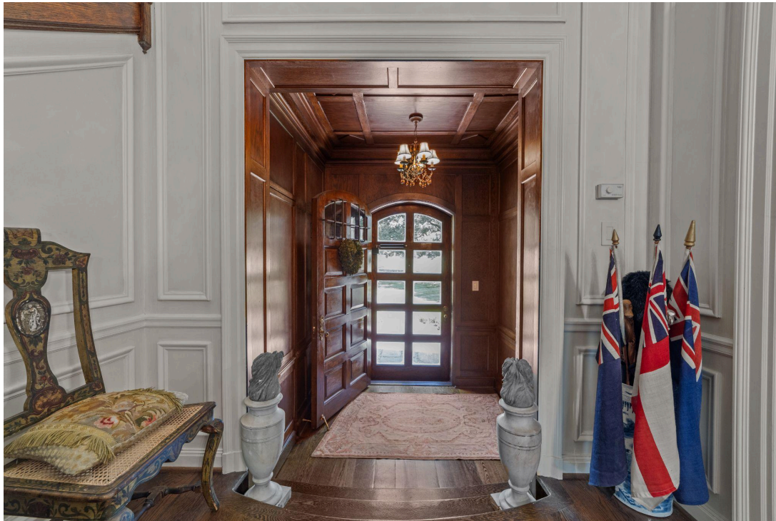
Image 27: Main entrance interior showing the interior side of the 10 lite solid wood door.
