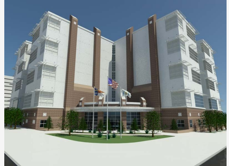
Guilford County Detention Center
