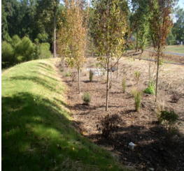
Bioretention Area at Summerfield Park
